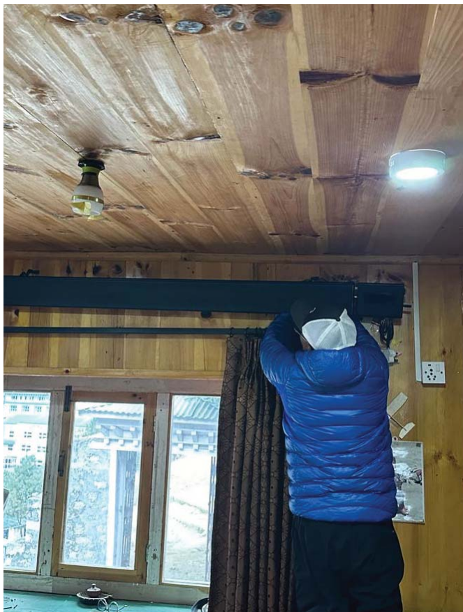
→ Wall heater, refrigerator and chair supported to Namche Dental Clinic.
